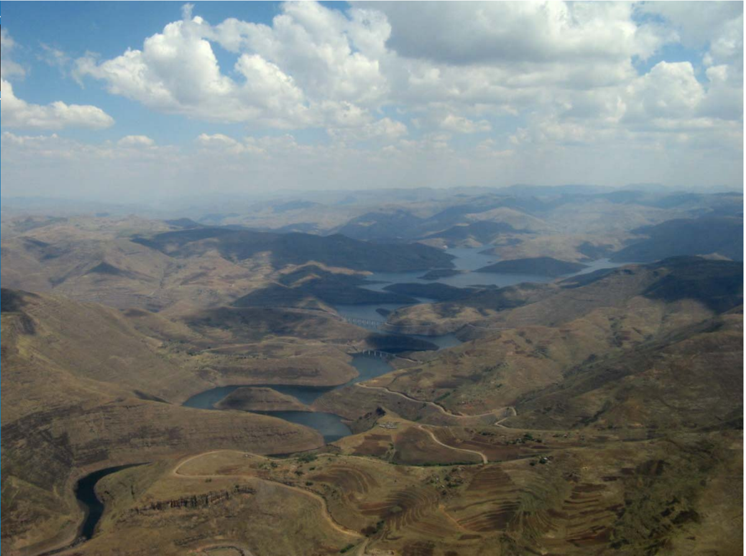
Existing major infrastructure: Mohale Dam reservoir
